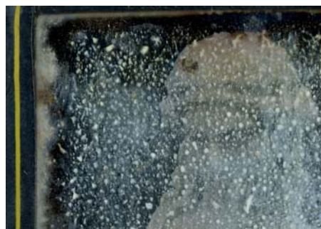
Fig. 77: Close-up of glass deterioration
